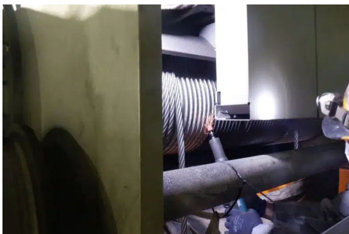
給電線改修 before
